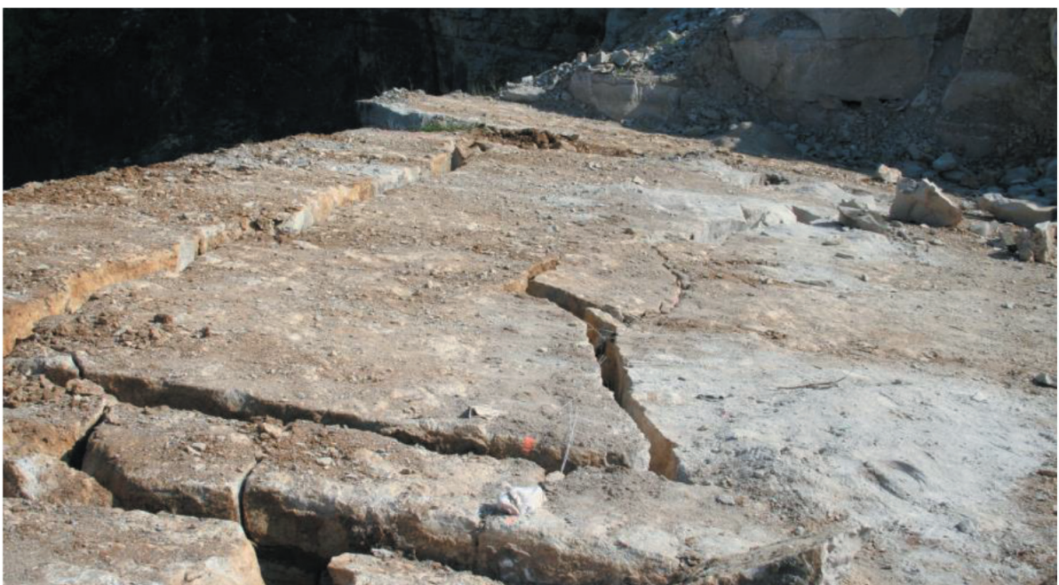
Rys. 11. Efekt urabiania ROCKSPLITTER-a Fig. 11. The effect after the ROCKSPLITTER blasting operations
