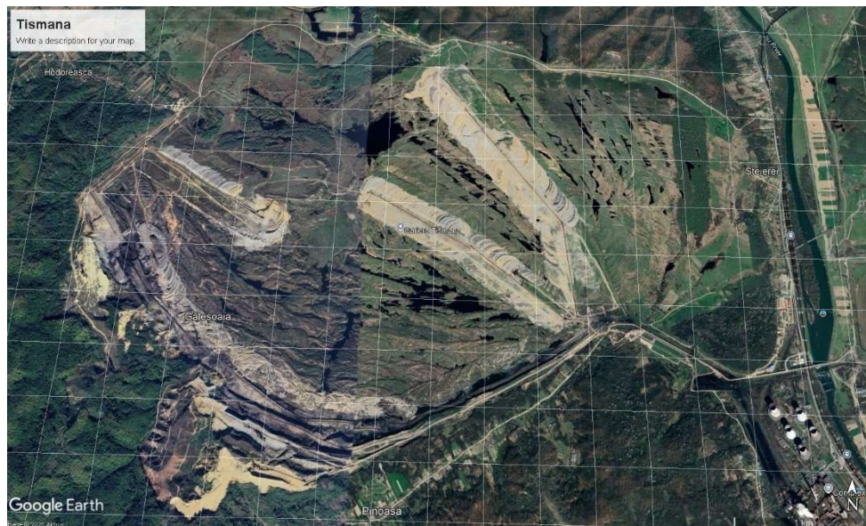
Fig. 27 Tismana open pit and internal waste dump (Google Earth Pro)
