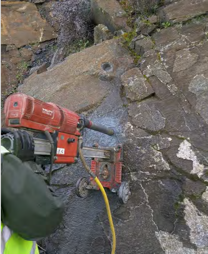
Core extraction process
