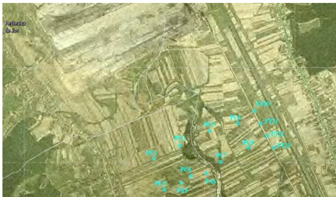
Location of dewatering drilling for groundwater from the phreatic aquifer and the Motru complex
