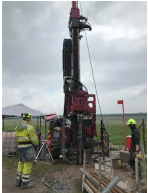
Sonic Drilling at project site
